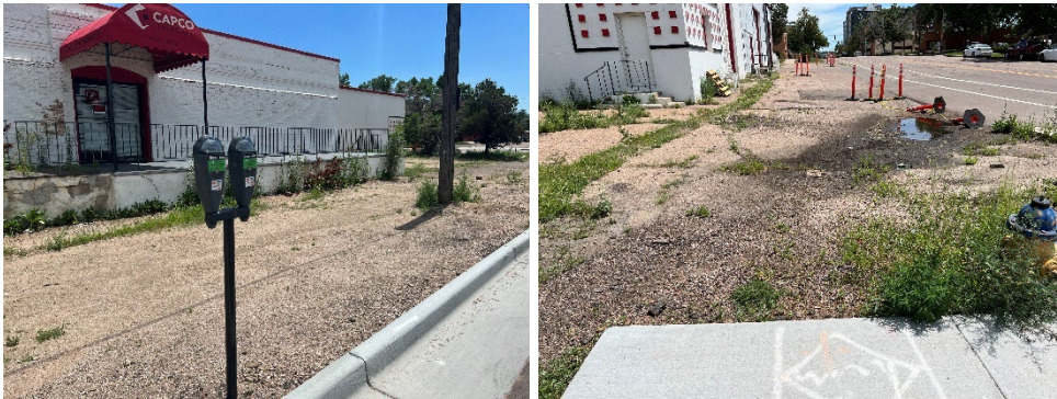
Figure 13. Lack of Sidewalks and Curb
