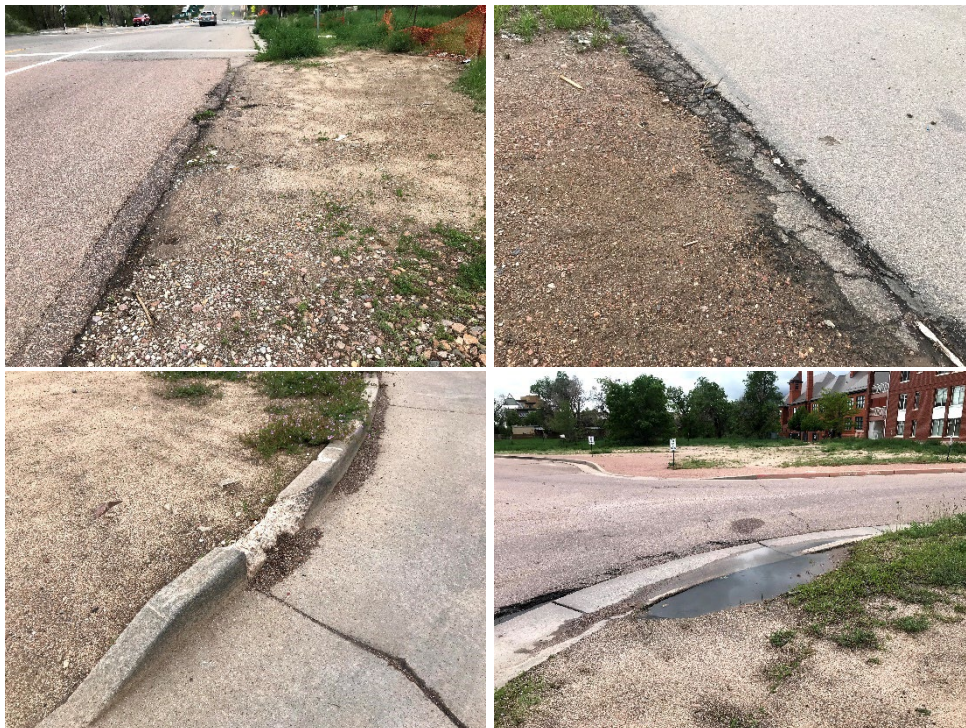
Figure 8. Deteriorated Curbs
