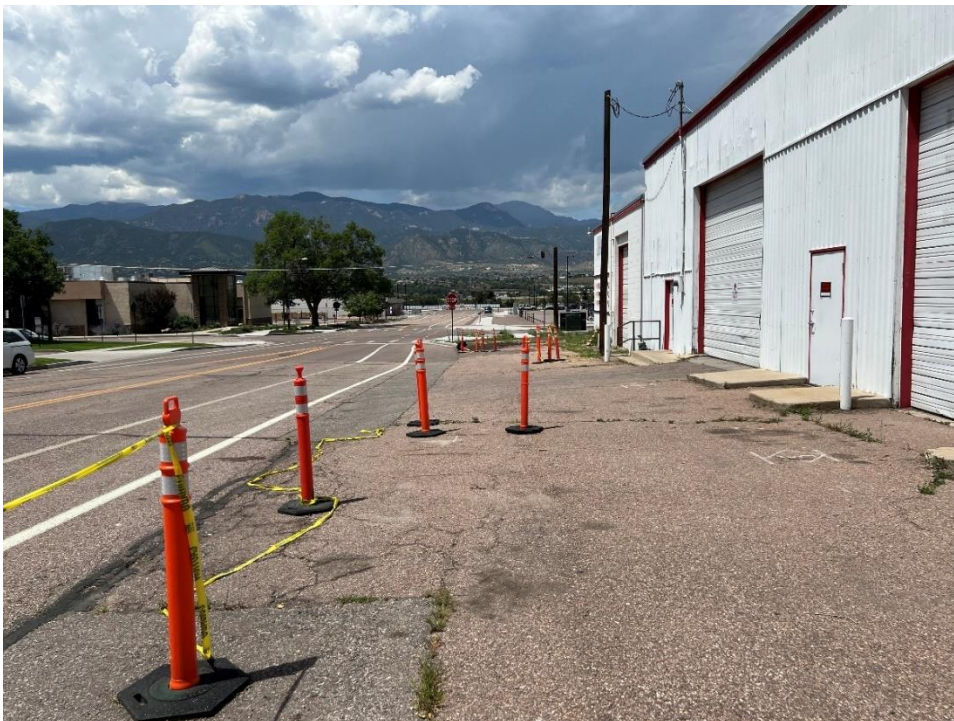
Figure 5. Excessive Curb Cuts Along Commercial Blocks
